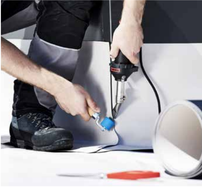
HOT JET S ideal for detail work on the roof.
