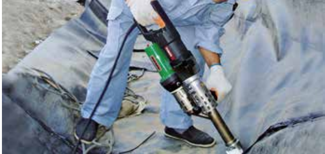
Due to its length, the FUSION 3 is especially suited for civil engineering applications.
